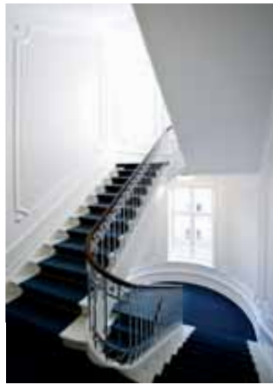
The beautiful old stairway from 1894 has been completely restored with great respect for the original. The stairway acts as the spinal chord of the house, reminding us that this is a fine old house with history.
